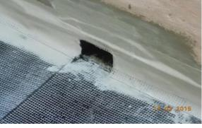
b) The laying of the waterproofing membrane, including the integration of horizontal sheeting with the vertical skirting water proofing and with the flanges of the side wall outlets (above) and the "wrapping at stairs and doorways (see below)
